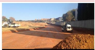
The service road is being repaired and resurfaced going up towards the 4 x 4 facility ending behind Leeukop corner.
