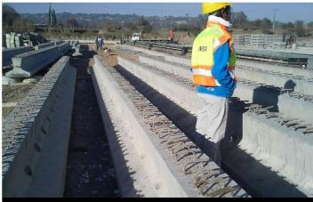
The beams for the underpass have been manufactured. They will be transported to site and placed over the underpass in mid July.
