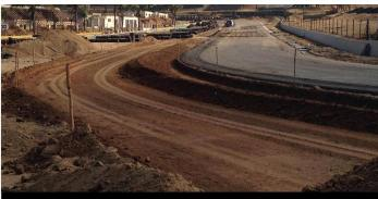
The run off area at Sunset being prepared. The gravel trap will have a section of tar run off as part of new safety upgrades.
